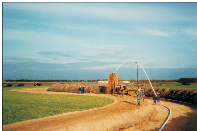
Fig. 4: Laying Aramid-Reinforced Plastic Pipes
